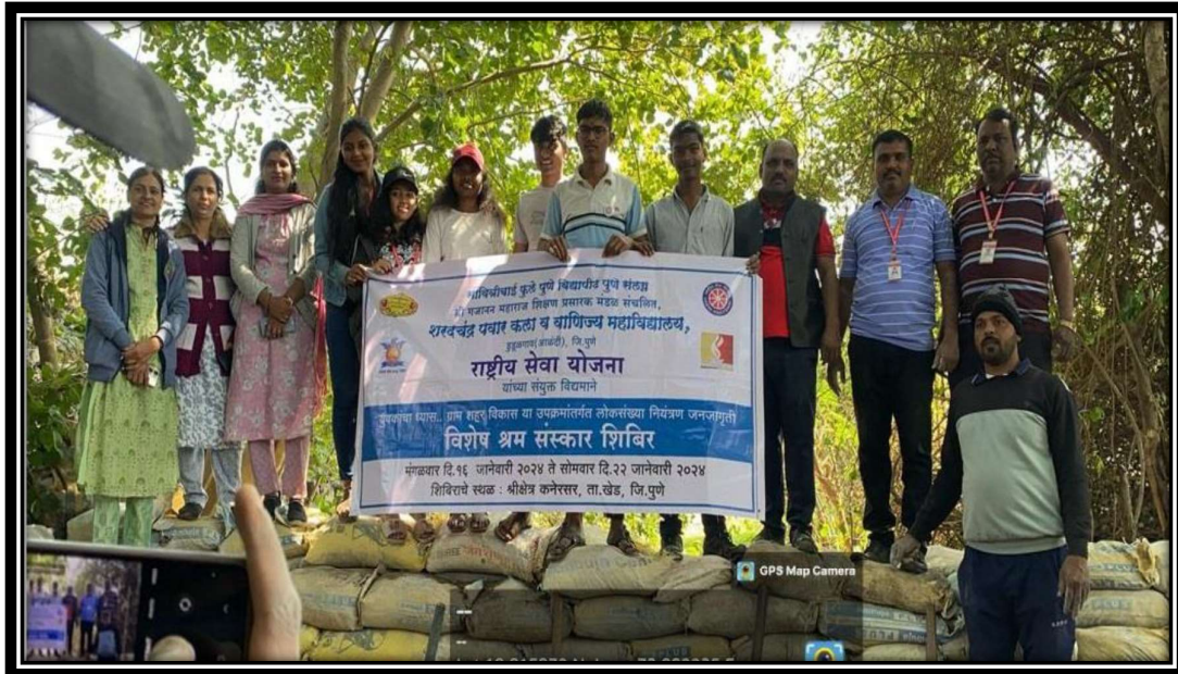
(Students built a dam in Kanersar Village)
