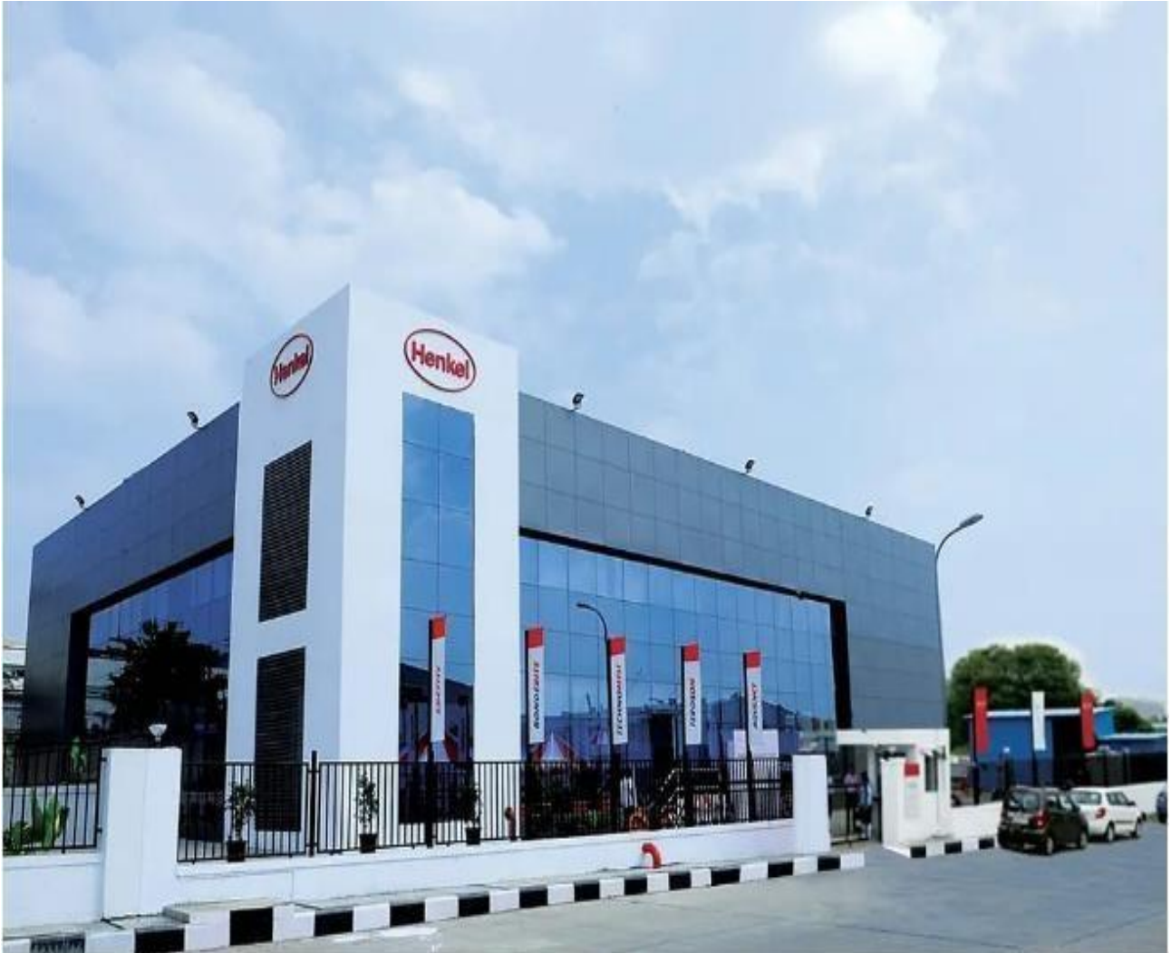
Henkel Pvt.Ltd. Kurkumbh, Industrial Visit Photographs
